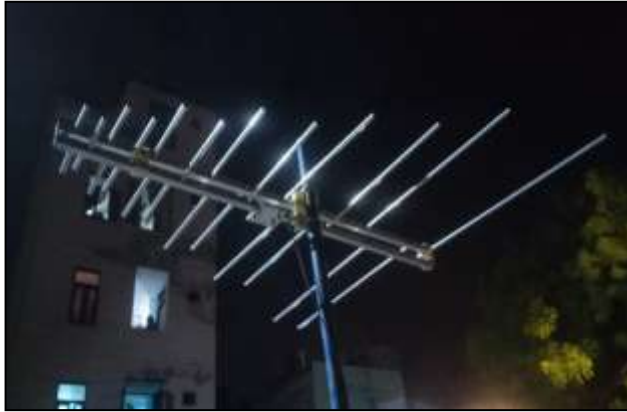
Frequency: 150~500 MHz / Gain: 9 dBi
